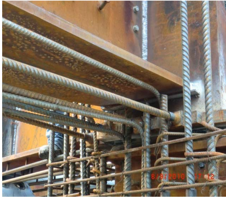
Photo 11 : Connection of composite beam and column structure
