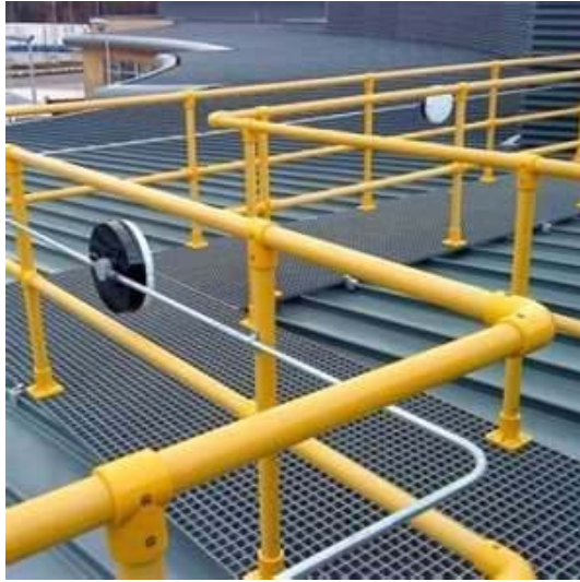
Photo 21 : Glass Reinforced Handrail
