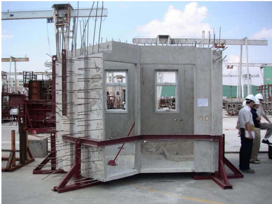
Photo 4 : Precast bathroom cum kitchen
