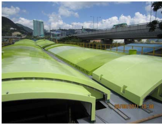
Photo 22 : Glass Reinforced Plastic Roof Panel
