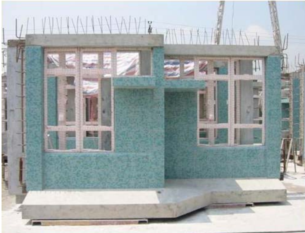
Photo 3 : Precast building façade with window frames
