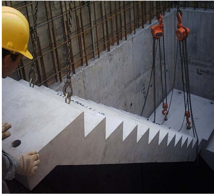
Photo 7 : Precast staircase
