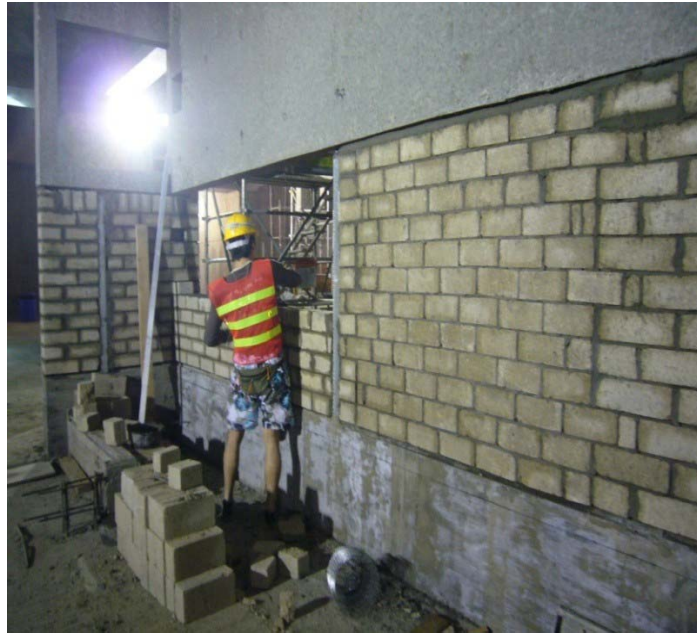
Photo 5 : Precast concrete block wall
