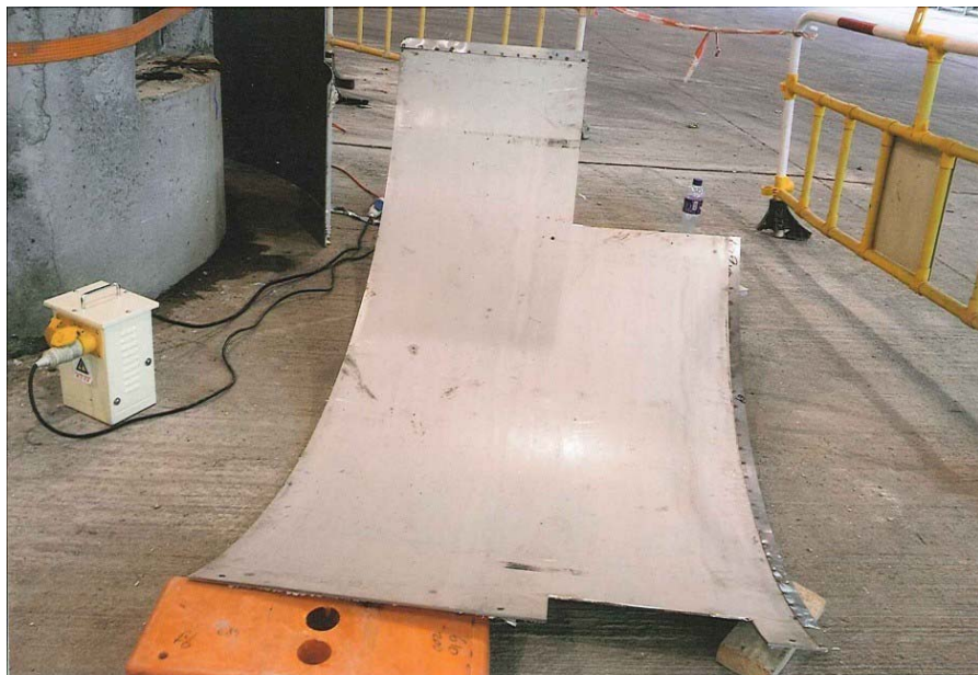
Photo 2 : Special design (curvatures) involving high workmanship requirements
