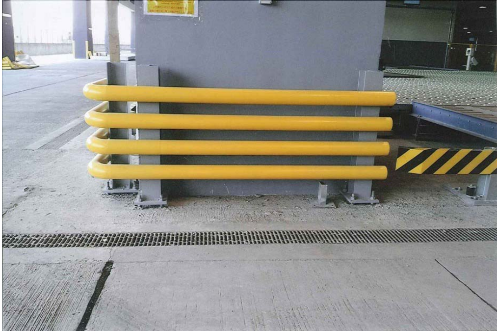
Photo 20 : Proprietary products to replace traditional welding in parapet installation
