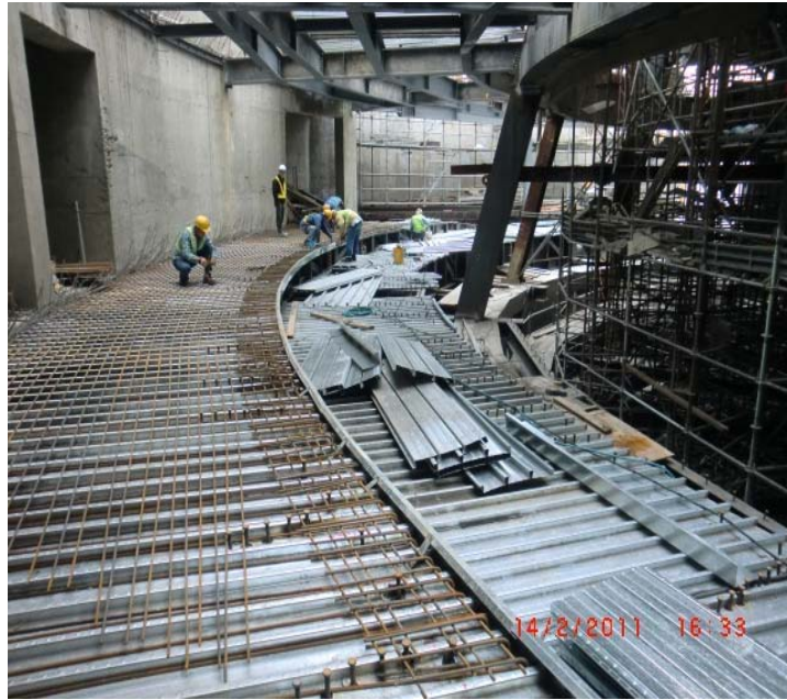
Photo 9 : Composite floor comprising steel and concrete structures
