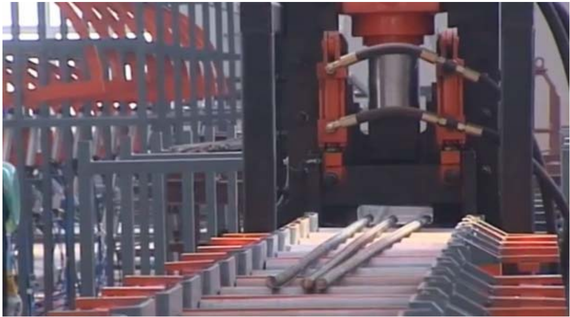
Photo 15 : Mechanical plant for cutting and bending of reinforcement bars
