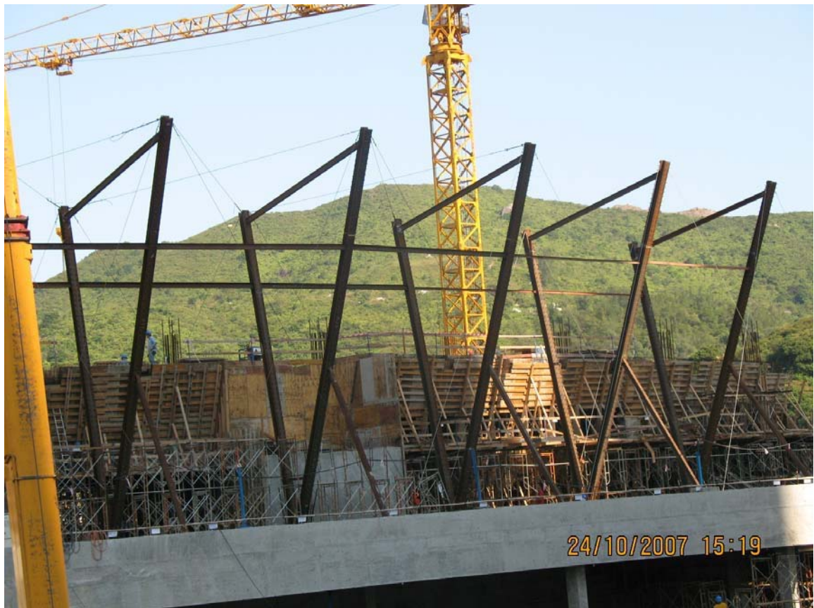
Photo 10 : Composite V-shaped columns for building construction
