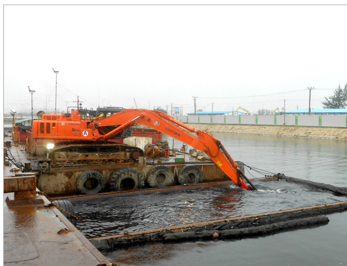
Figure 4 Excavation of sediments using close grab mounted on flat top pontoon
