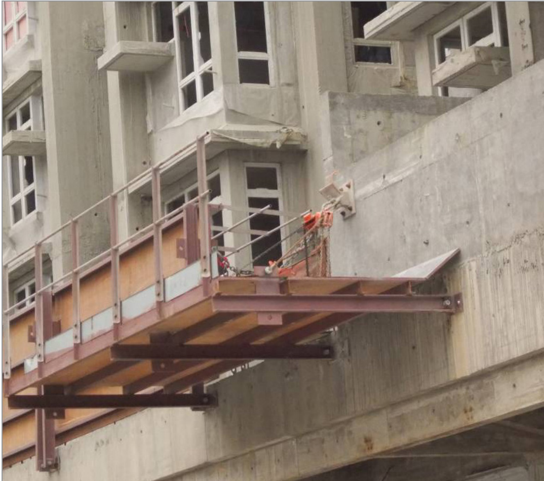
Figure 15 Temporary Protective Canopy used in the construction site
