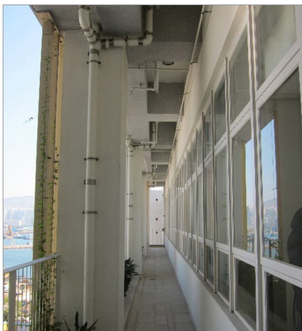
Figure 3 The view of Maintenance corridor
