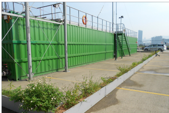
Figure 7 Provision of earth bund surrounding the chemical storage yard
