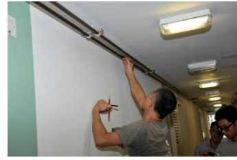
3. Marking direction of flow on pipe body before dismantling
