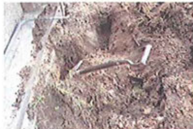
AG Root Excavation Along Wall South of Tree
