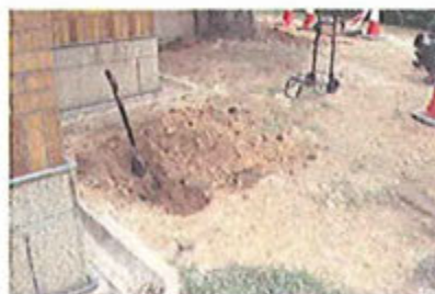
Trench 2 – Test Pit Dug by AG to Identify Cut Roots
