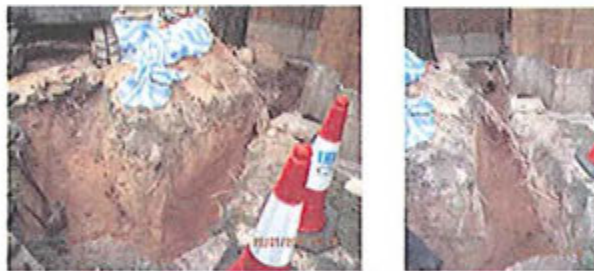
Photos of Trench 1 Provided to AG by LCSD
