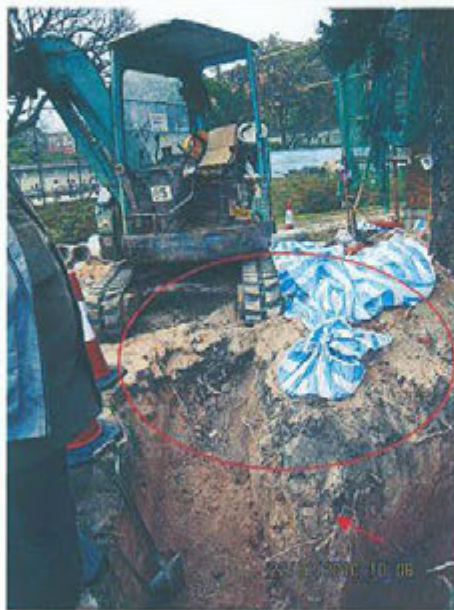
Fig 9. Heavy duty machine on surface, record on Jan 23.
