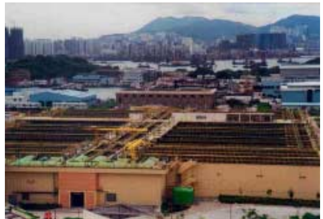
Figure 6 - Sedimentation Tanks Facilities
