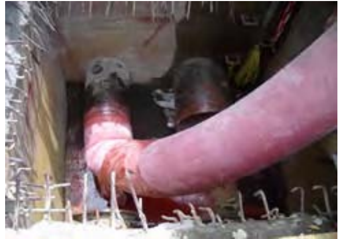
Figure 3: Steam Curing of CIPP
