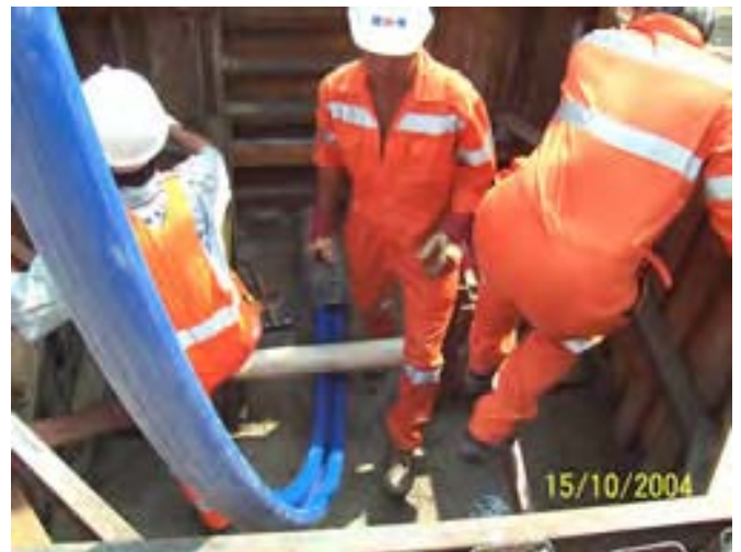
Figure 6: Pre-fold Liner Method in Progress
