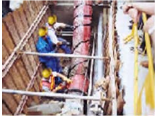
Figure 2: CIPP Installation in Progress
