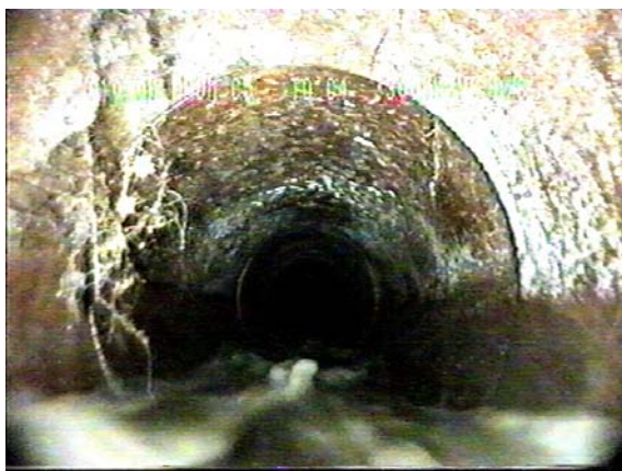
Plate F11 Roots of Less Than 10 mm Thick
