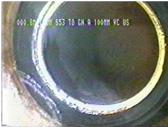
Plate F7 Open Joint Displaced over 1.5x Pipe Wall Thickness
