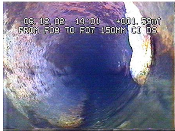
Plate F14 Deposition of Dissolved Salt on Pipe Wall
