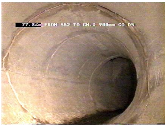
Plate F17 Line Deviation of Pipe to the Right
