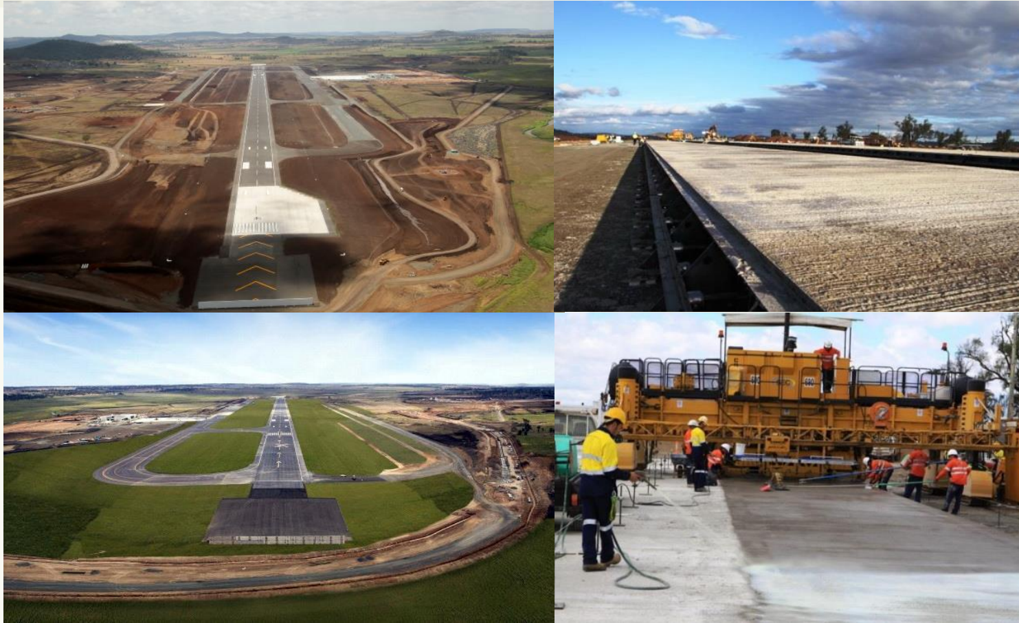
Airport pavement built with in-situ AAM concrete
