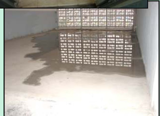
Inadequate fall gradient
