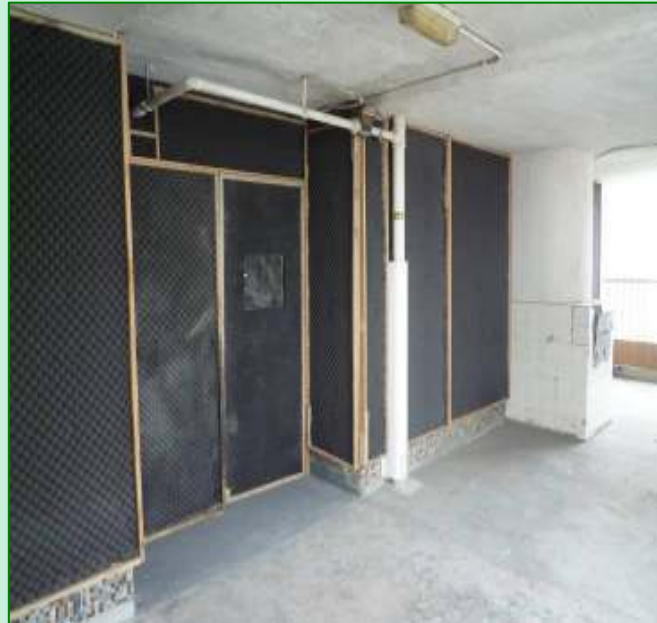
Noise Absorbent Curtains at working areas to reduce noise and dust
