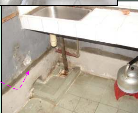
Undesirable Drain Design
