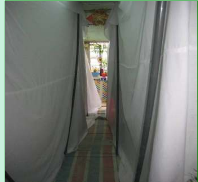
Dust Screen Protection in Tenant's Flat
