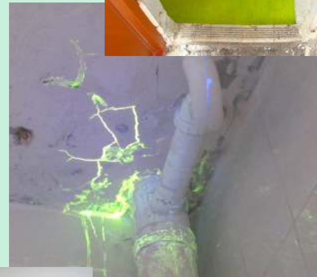
Use of Florescence Solution for Seepage Detection
