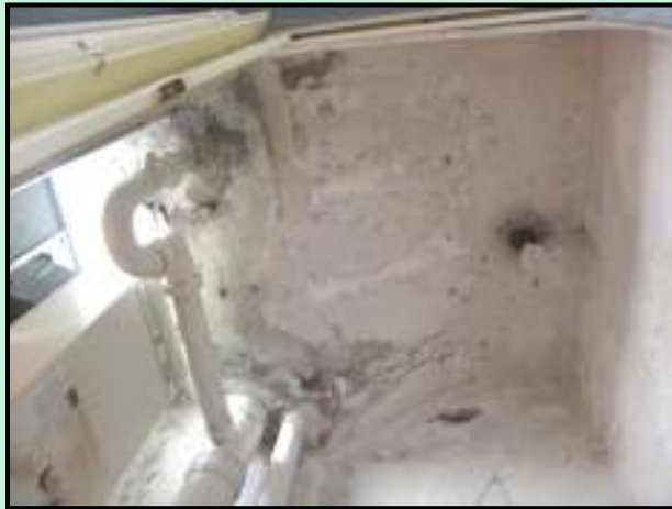
Piping Through Slab
