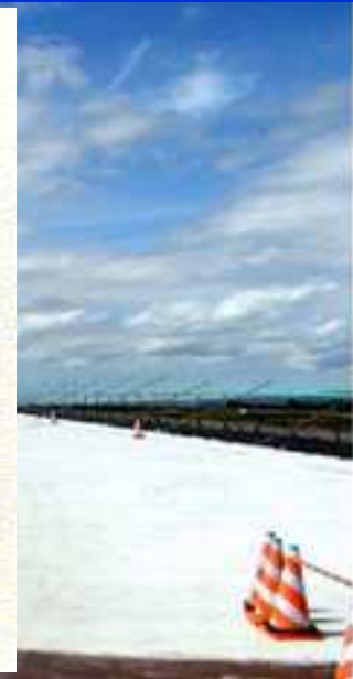
Self-Flow PDCC placed on top of Steel Section for Mihara Bridge
