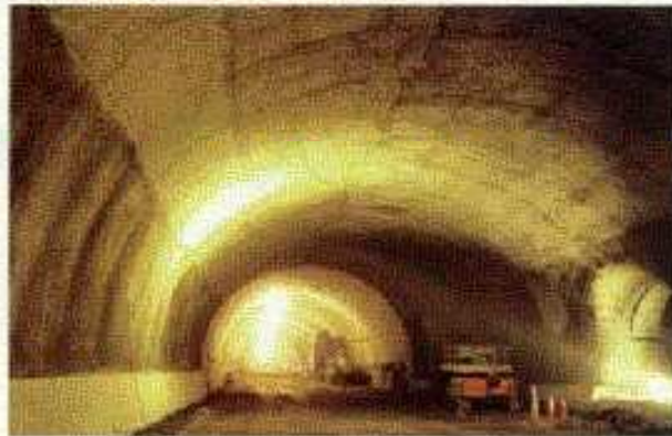
Sprayed PDCC Lining for Hida Tunnel
