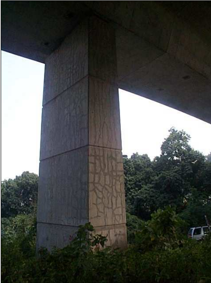
Map Cracking on concrete column – ASR
