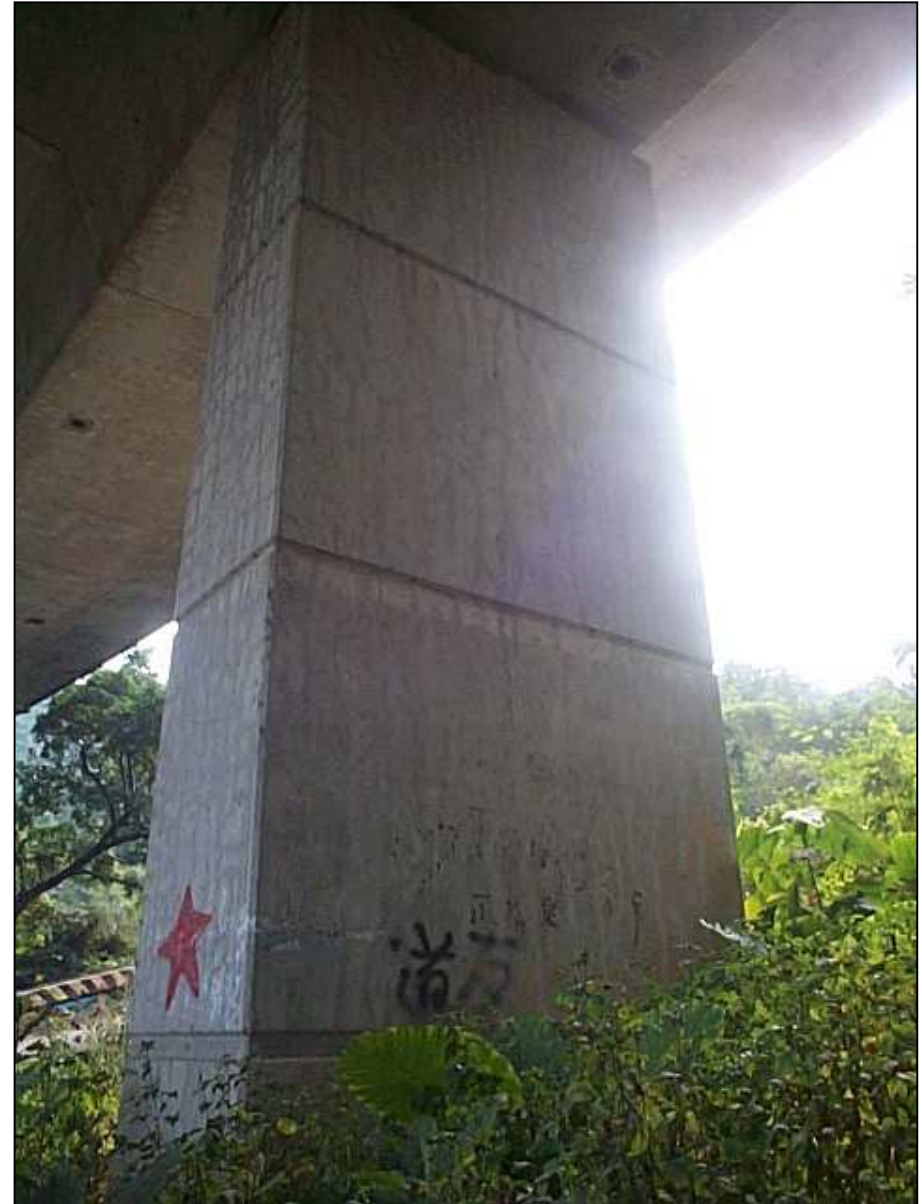
Map Cracking on concrete column – ASR
