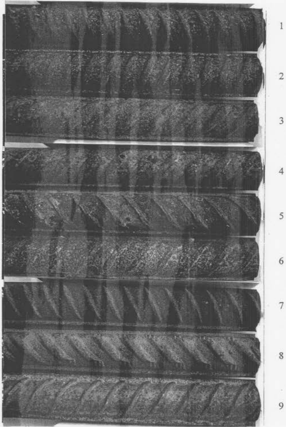
Plate 50 - Rust Guide for Steel Reinforcement Bars Nos. 1-6 : not acceptable; Nos. 7-18 : acceptable (From App. 15-A. General Specification for Civil Engineering Works, Guidance Notes, 1992)
