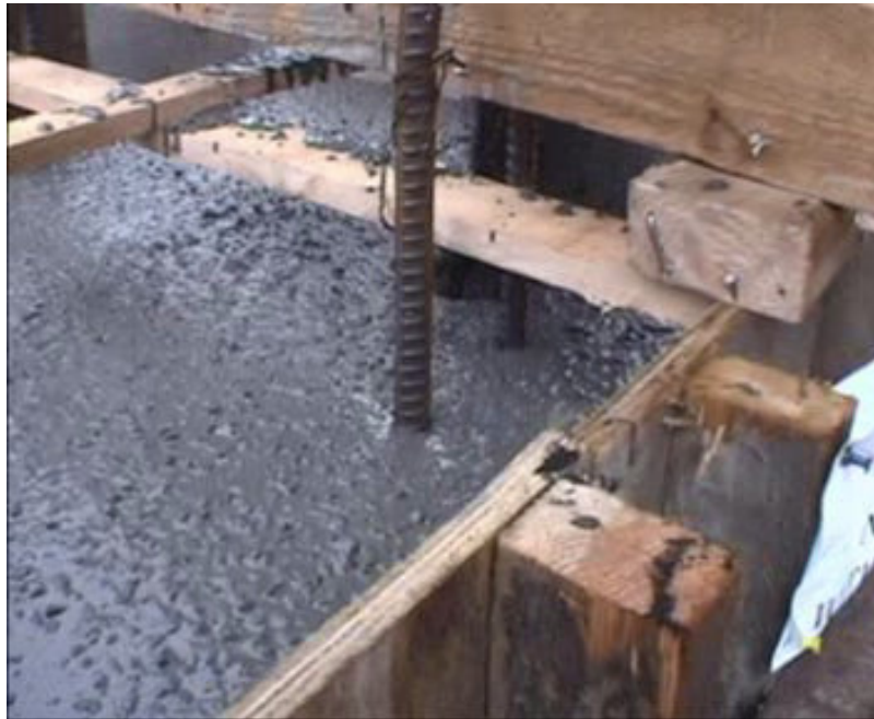
Trial Block – Casting of SCC into Formwork
