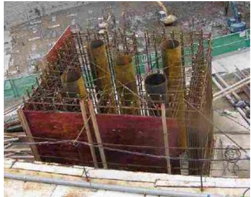
Trial Column Construction
