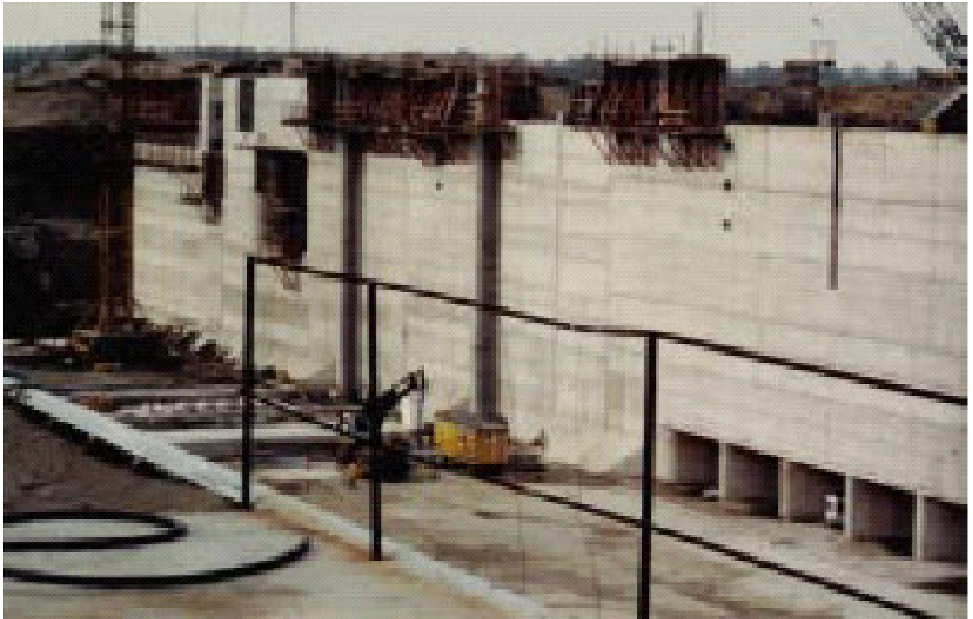
Berendrecht Lock in Belgium 1987-1988 (C 35 recycled concrete)
