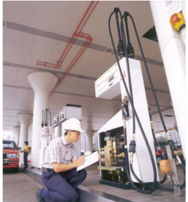
Photo 2 - LPG Filling Station
