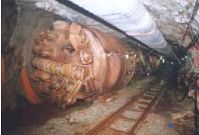
Figure 3 - Tunnel Boring Machine (TBM)
