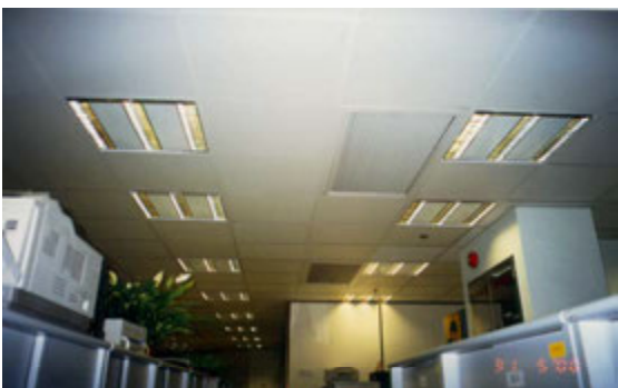
Fig. 10 Lighting after retrofit with new T5 luminaires
