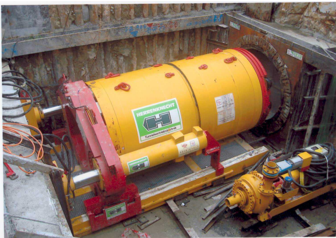
Photo 4: A Tunnel Boring Machine in a jacking pit
