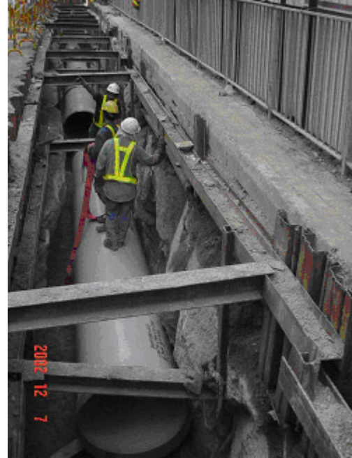
Photo 1: Mainlaying of 1,000 mm fresh watermain along along Fu Mei Street
