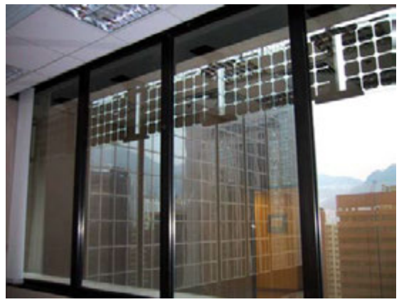
Figure 3: Sunshade Type Sub-system (Interior view)
