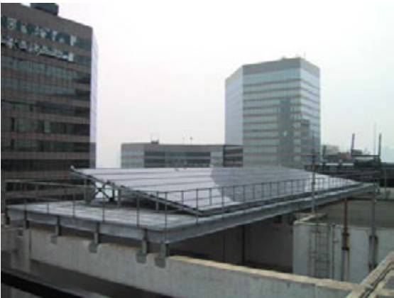
Figure 2: Rack Type Sub-system
