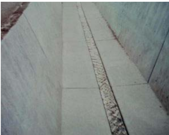
Figure 3 : Catchwater channel after repair
