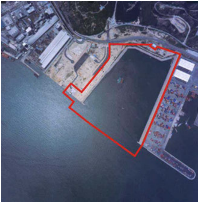
Figure 1 – Aerial photos showing Tuen Mun Area 38 Stage 2 Reclamation
