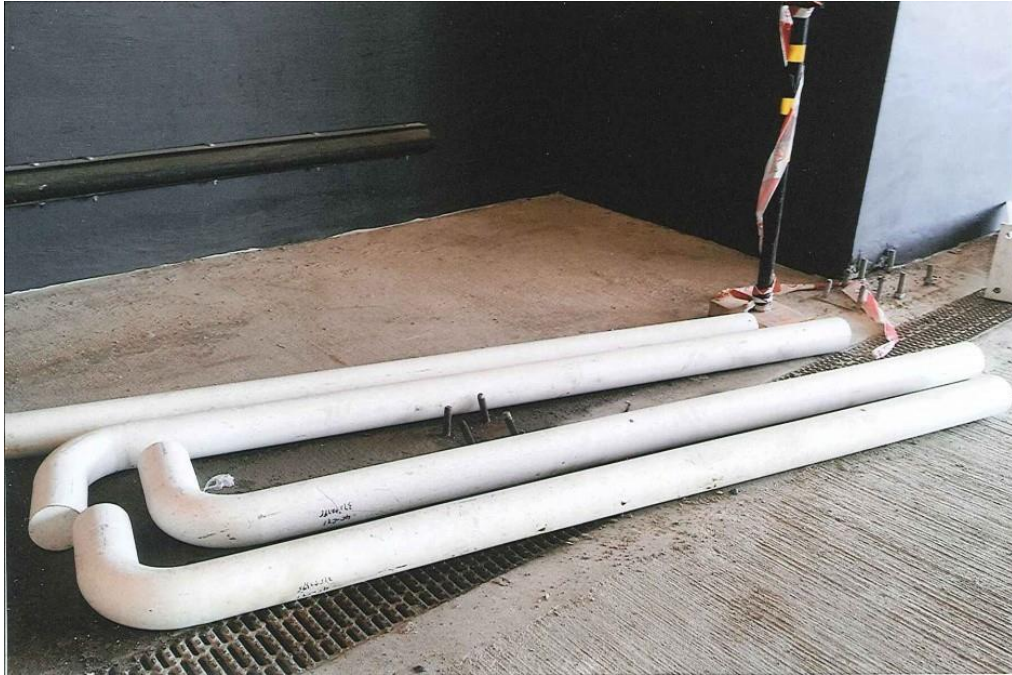
Photo 19 : Proprietary products to replace traditional welding in parapet installation
