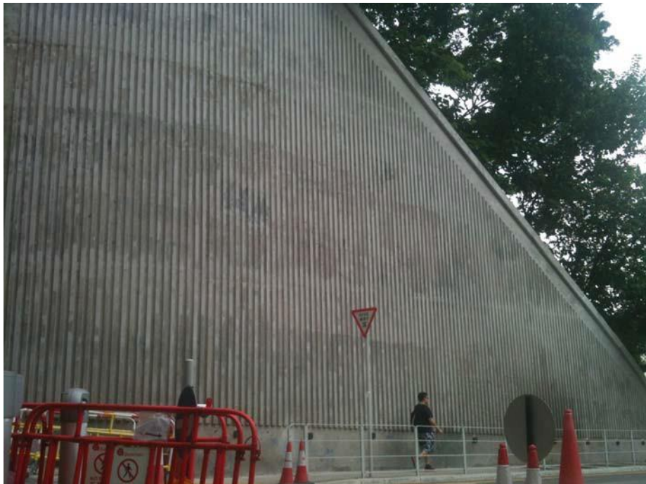
Photo 18 : Profiled finishes on the external faces of retaining walls to be avoided
