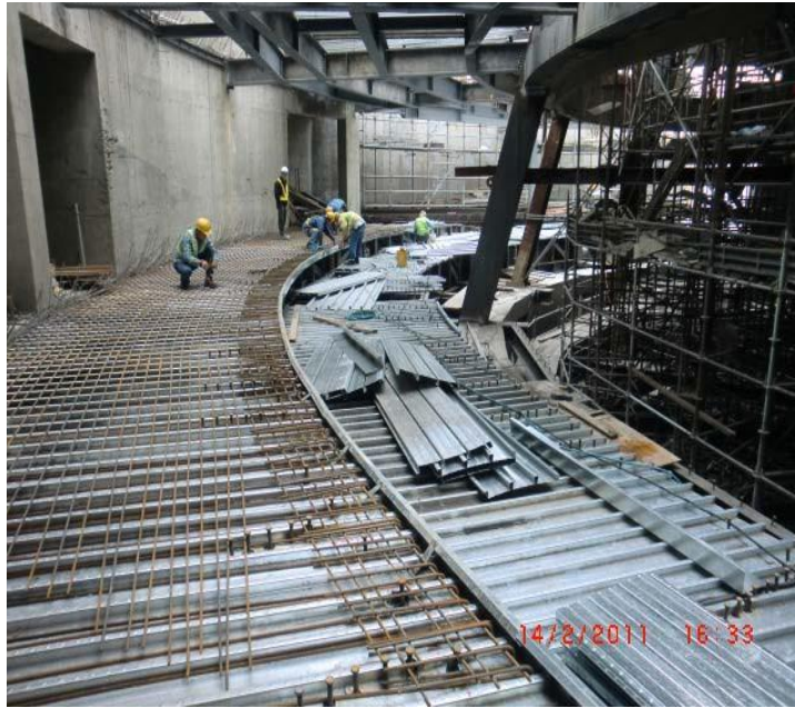
Photo 9 : Composite floor comprising steel and concrete structures
