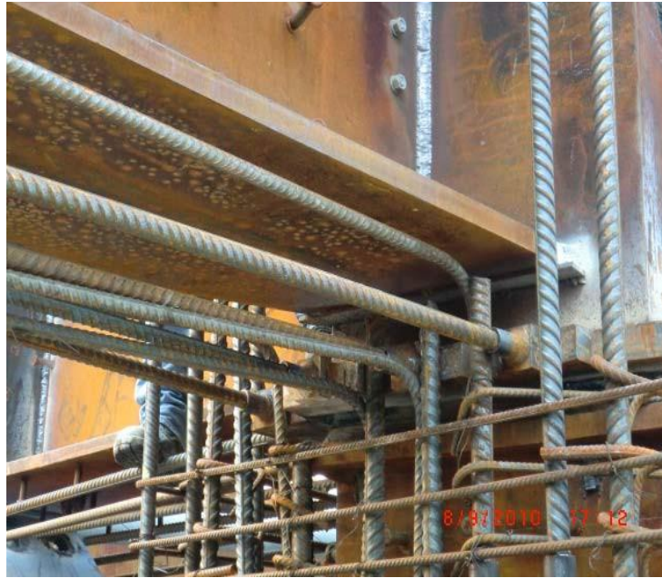
Photo 11 : Connection of composite beam and column structure
