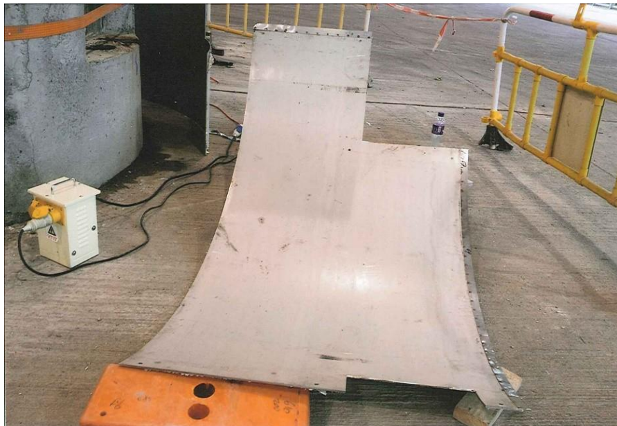
Photo 2 : Special design (curvatures) involving high workmanship requirements
