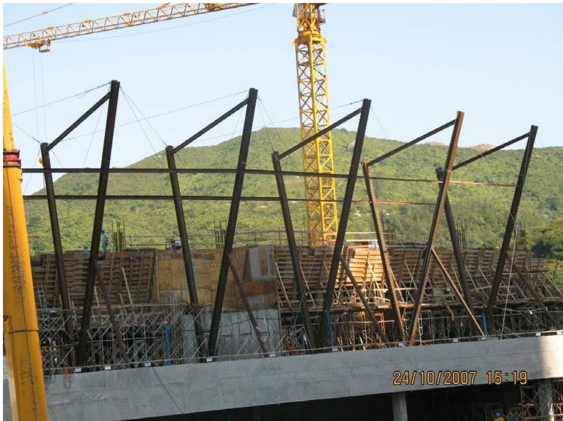
Photo 10 : Composite V-shaped columns for building construction
