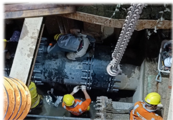
④ Workers meticulously tightened every screws and repeatedly inspected connection points, ensuring every detail is perfectly 'spot on'. (DC/2018/06)
