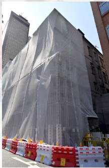
Erection of scaffolding at busy Gloucester Road side
