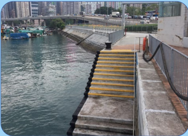
Construction of landing steps
