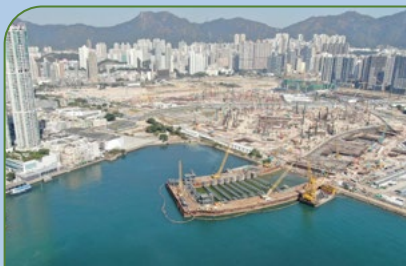
Temporary reclamation of CKR - Phase 1 (November 2019)
