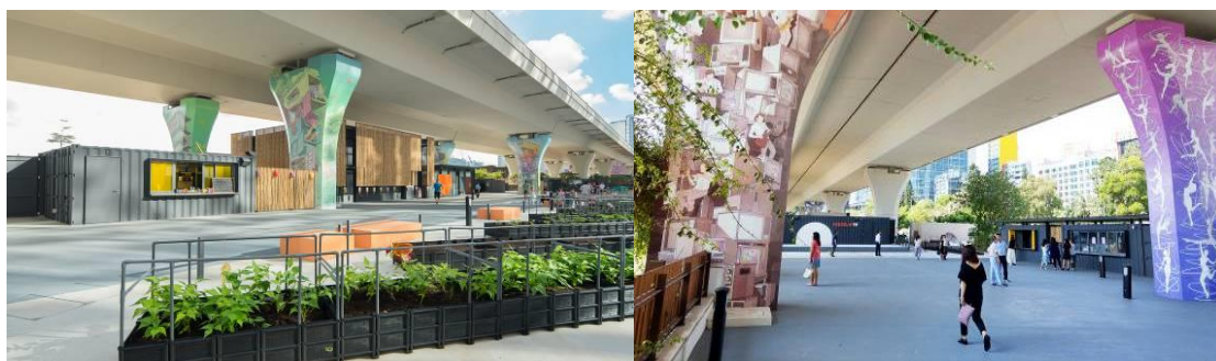
Fly the Flyover and Operation beneath Kwun Tong Bypass
