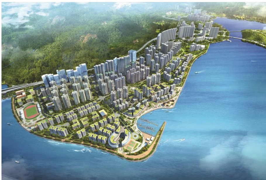
Tung Chung East Extension
