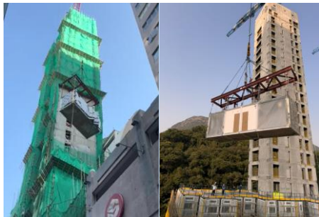
Modular Integrated Construction Method
