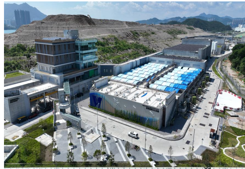
Tseung Kwan O Desalination Plant
