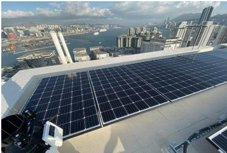
PV panels on the top roofs of residential towers
