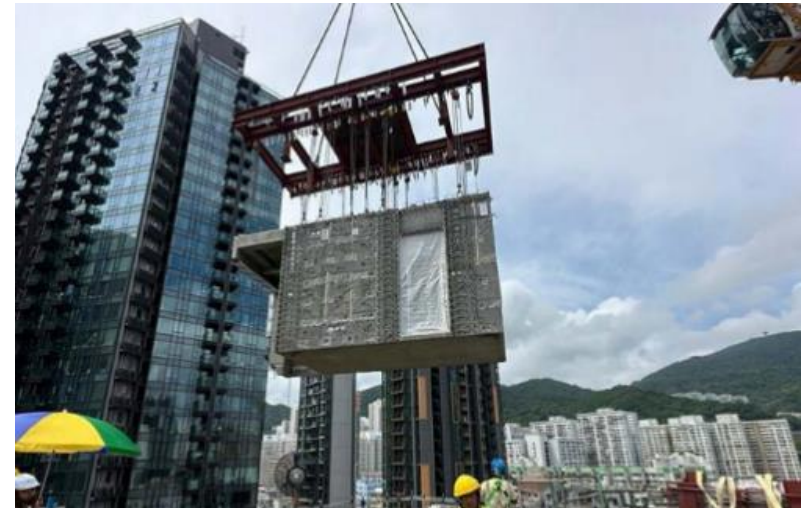
Modular Integrated Construction for SSP-015
