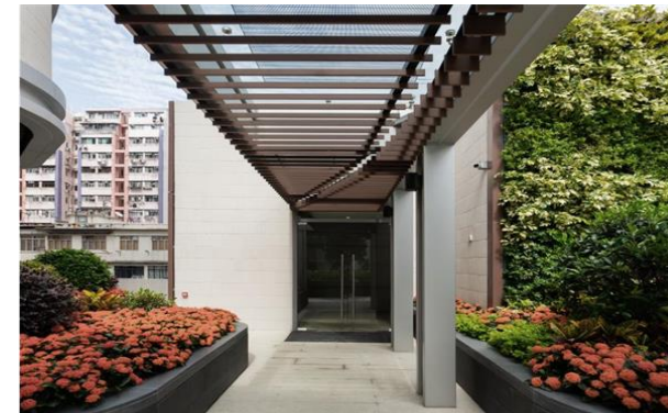
Building-integrated photovoltaics (BIPV) panels on 3/F Covered Walkway
