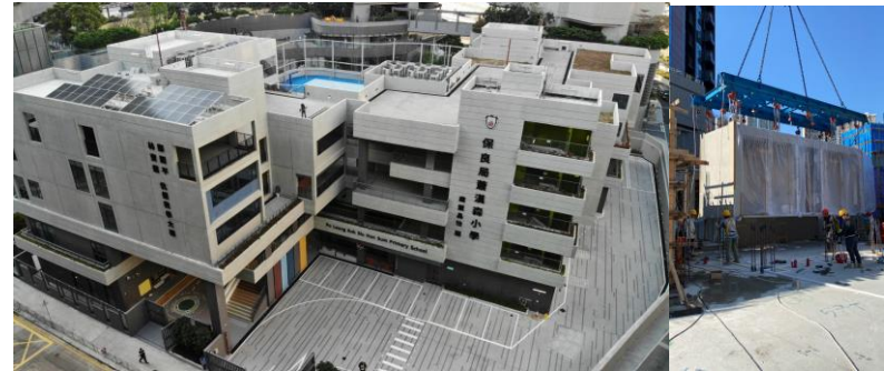
Modular Integrated Construction Method
