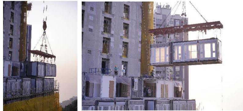
Modular Integrated Construction Method
