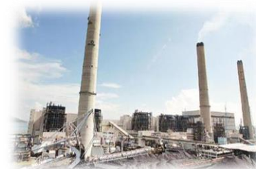
HKE - Lamma Power Station
