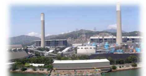
CLP - Castle Peak Power Station
