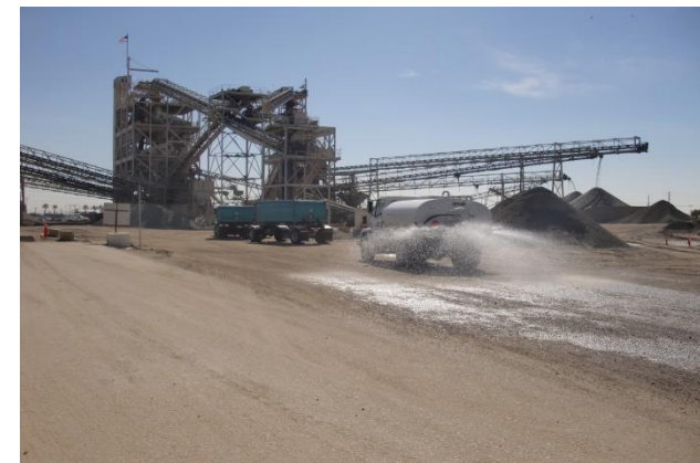
Open area dust control
