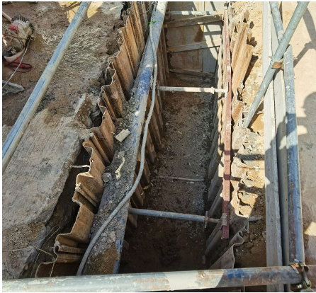
Trench before backfilling size: 4.0m*1.16m*2.3m
