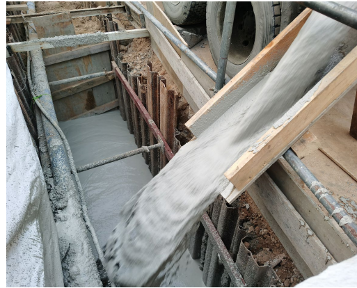
Filling with NAMI backfill materials
