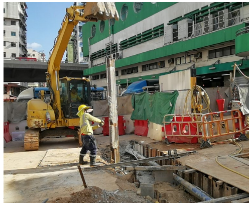
Removing sheet piles
