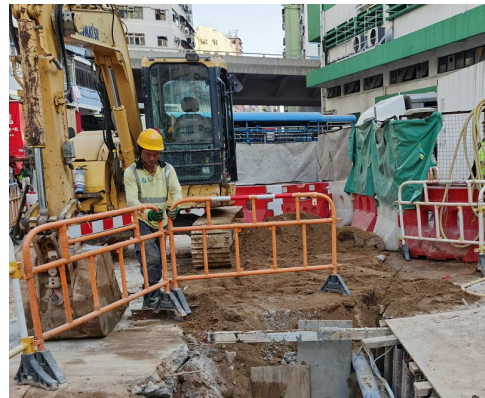
Filling the subbase
