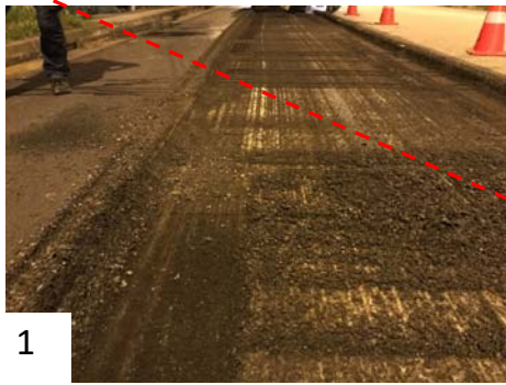
Mill off top asphalt
