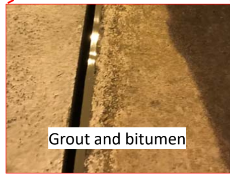
Grouting and sealing
