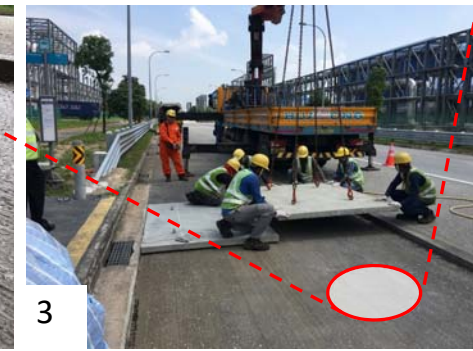
Place the slabs
