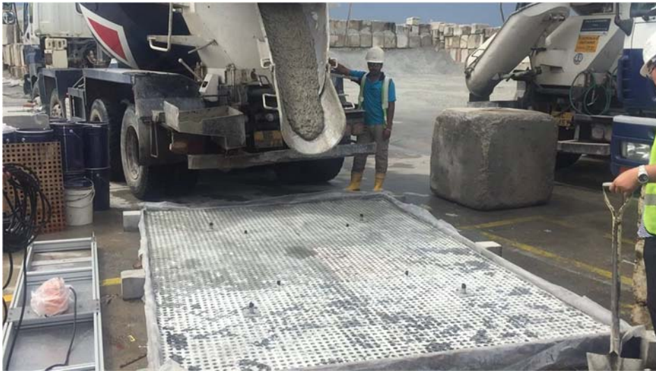
Casting ECC slab
