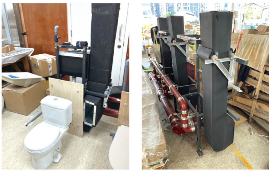
A 坐廁合成構件 MiMEP of closet (即已安裝排氣管道、給排水管道、鋼架中的傳感器) (i.e. completed with exhaust air duct, drainage pipework and water pipework, sensors in a steel rack)
