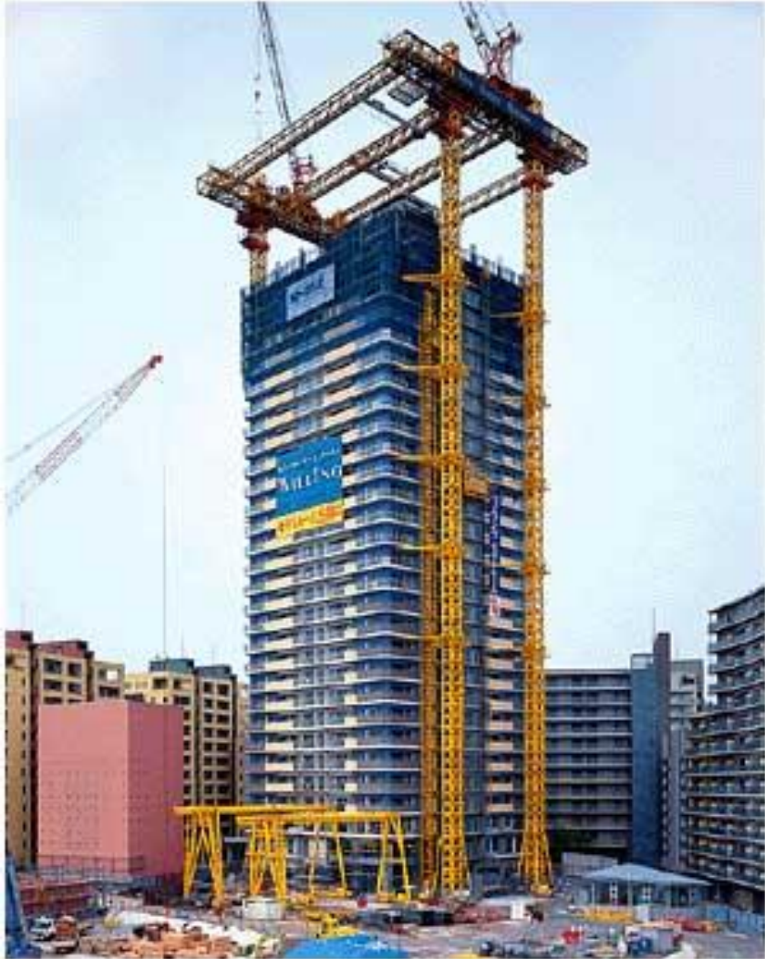
Robotized Construction SMART Automated Construction, SHIMIZU Co. Ltd.
