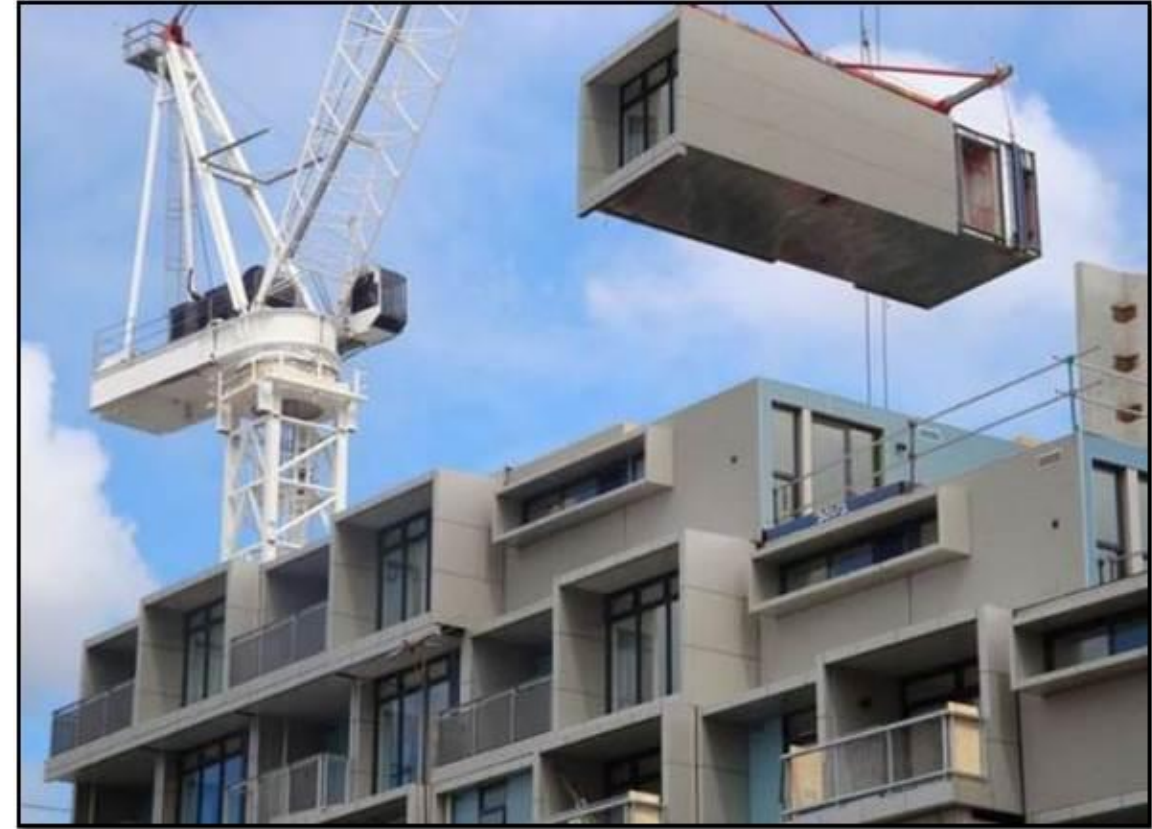
Modular Integrated Construction
