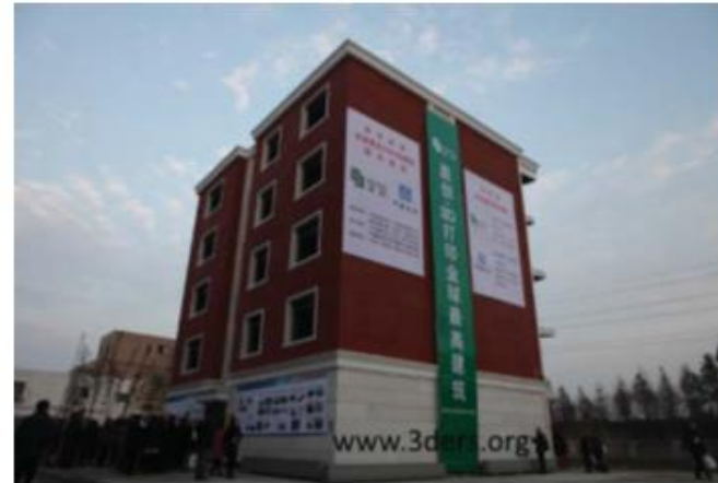
A 3D printed five-story apartment block (Charron 2015)
