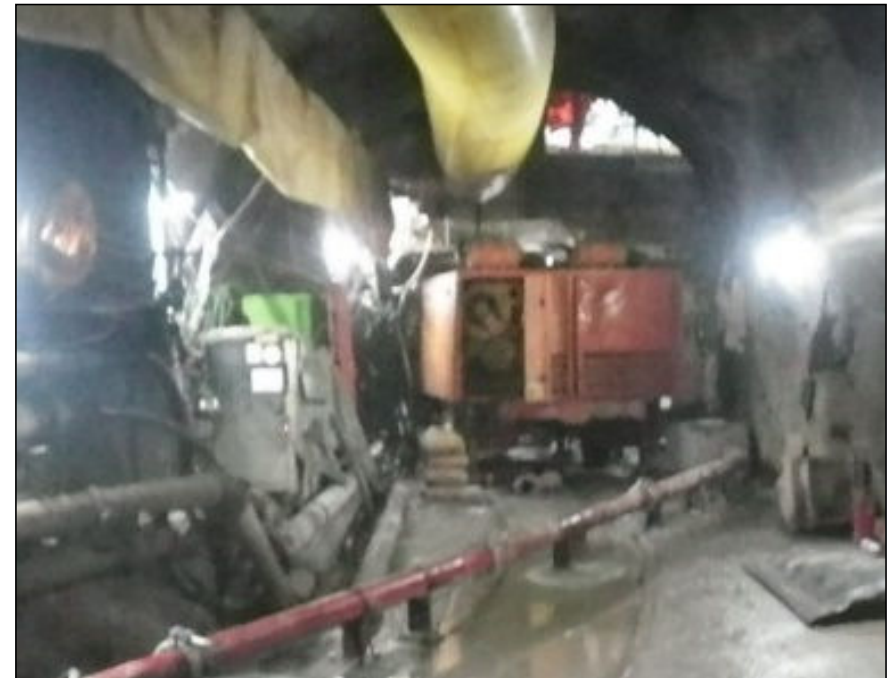
Concrete Pump at Shaft Bottom
