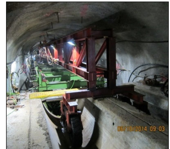
Formwork Carrier with Invert Formwork
