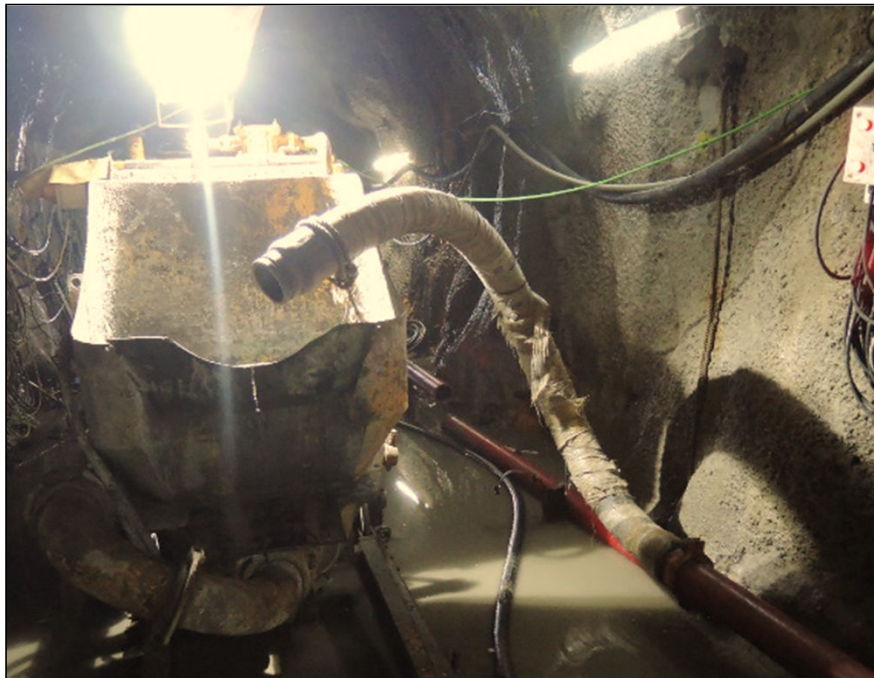
Concrete Pump at Formwork
