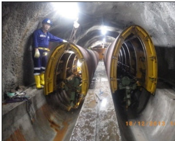
Vault Formwork
