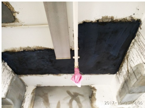
Ceiling at 2/F
