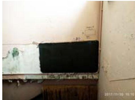
Beam on 2/F
