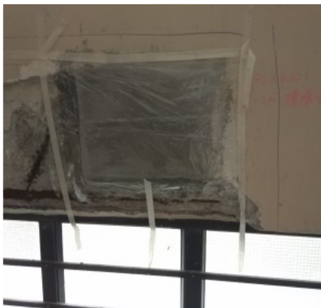
Below windows of staircase
