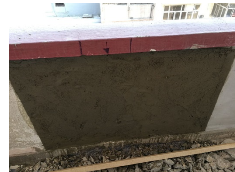
Parapet along the corridor
