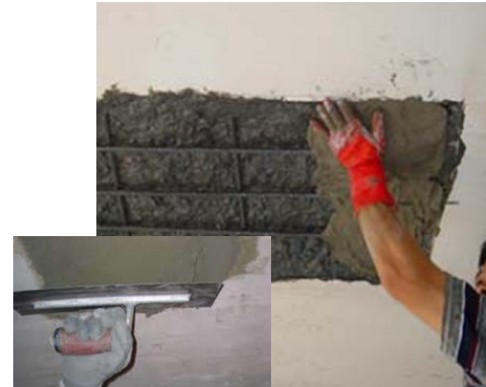
Typical Repair Location
