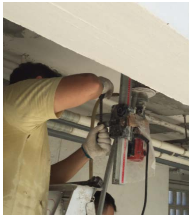
75mm dia. core containing full thickness of the repair
