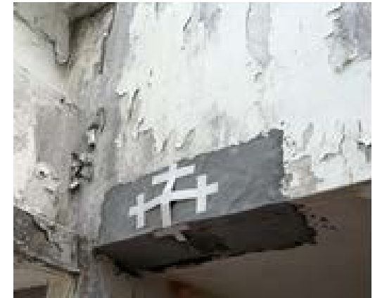
Wall at the outdoor roof
