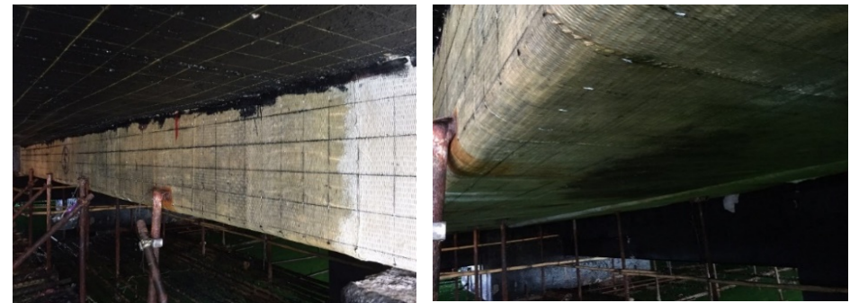
Location 2: Beam side and soffit
