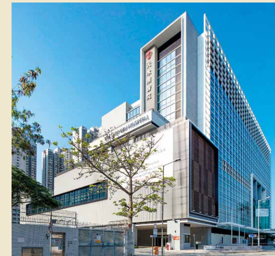
Design-and-Build Project – Tin Shui Wai Hospital
