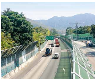
Retrofitting of Noise Barriers on Fanling Highway
