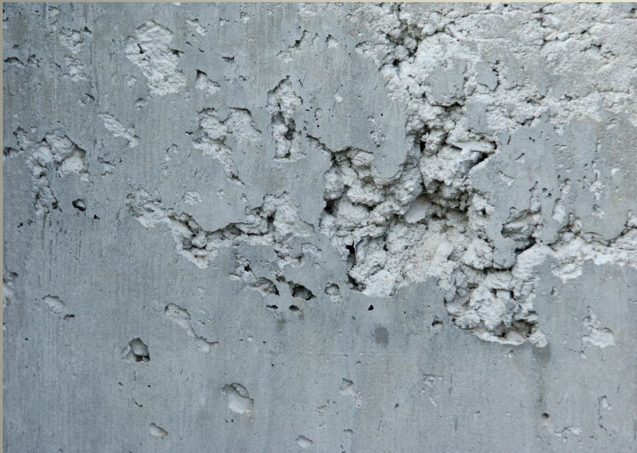
Inadequate Vibration - Honeycombing
