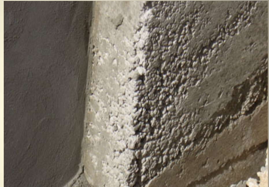
Inadequate Vibration - Honeycombing
