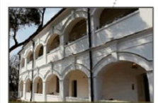
9 舊大澳警署 Old Tai O Police Station
