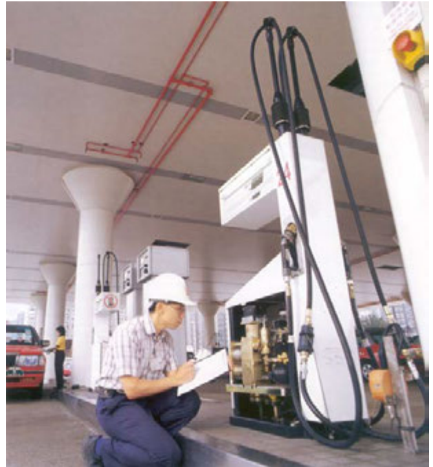
Photo 2 - LPG Filling Station
