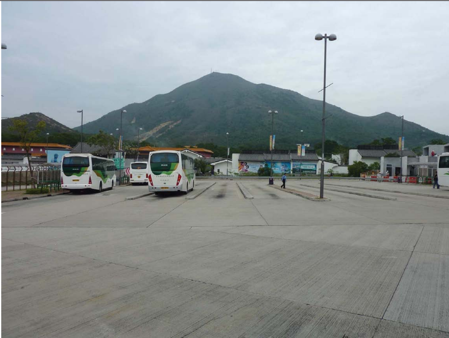
Annex 7 Ngong Ping Public Transport Interchange Photo 2
