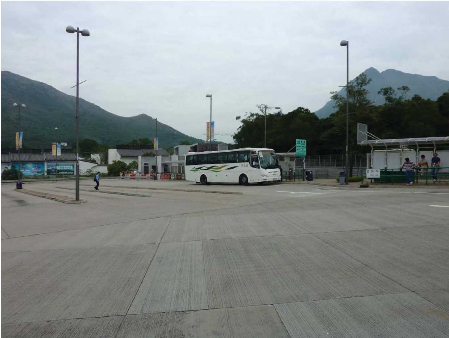
Annex 6 Ngong Ping Public Transport Interchange Photo 1
