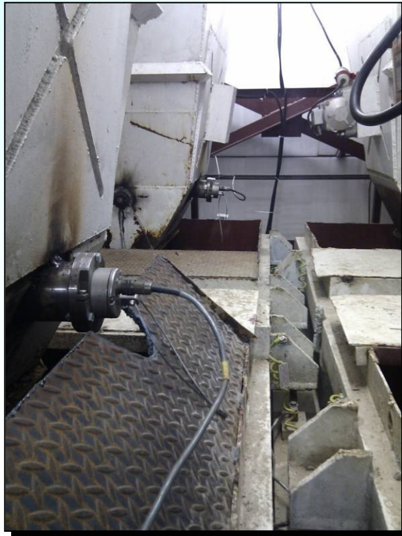
Probe Installation for 10mm / 20mm
