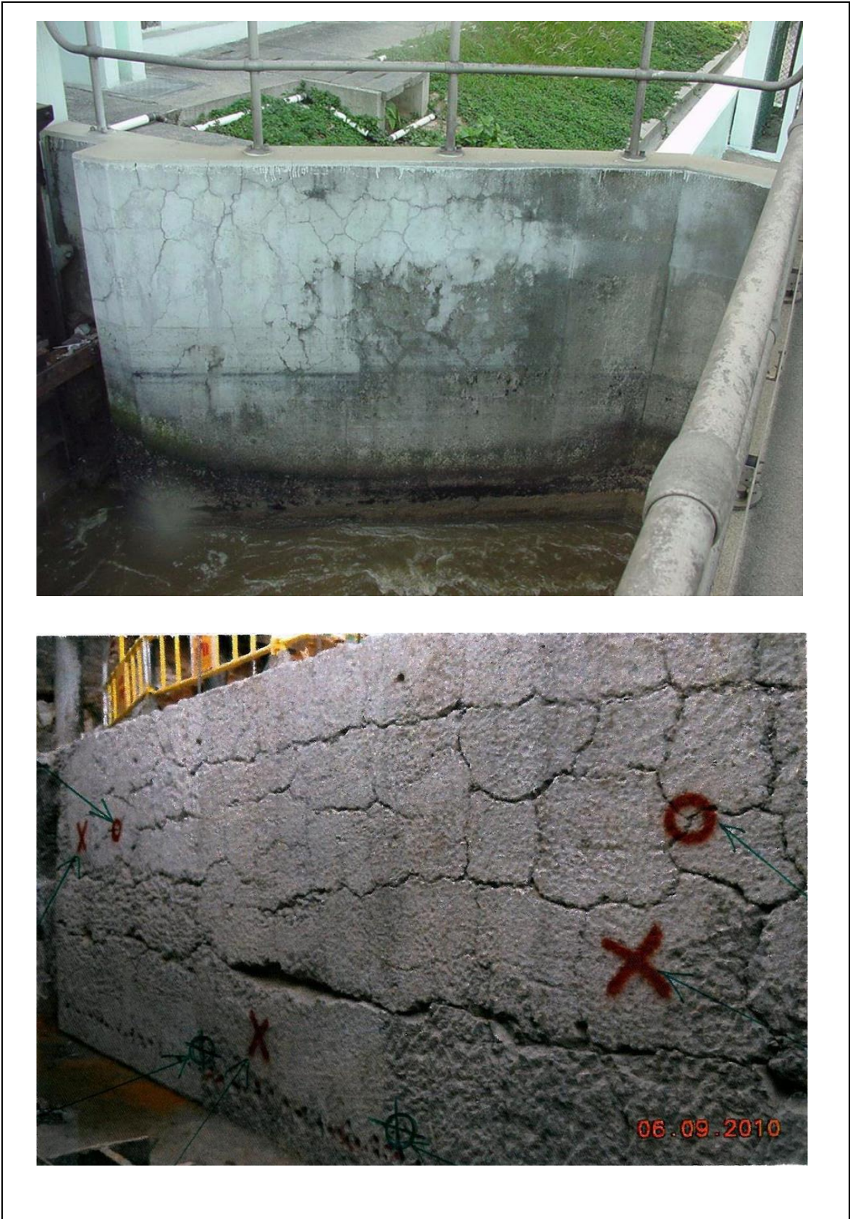
Figure 2.1 Typical Pattern of ASR Cracks
