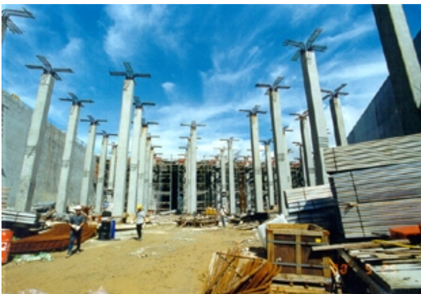
Butterfly Valley Primary Service Reservoir Stage I Project – Compartment Under Construction
