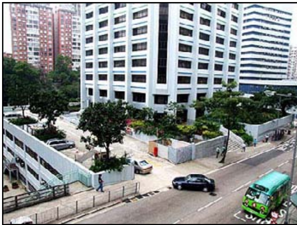
6.5 – Podium Garden, CEDD HQ, Ho Man Tin (Kowloon City District) (Source and copyright © by CEDD)
