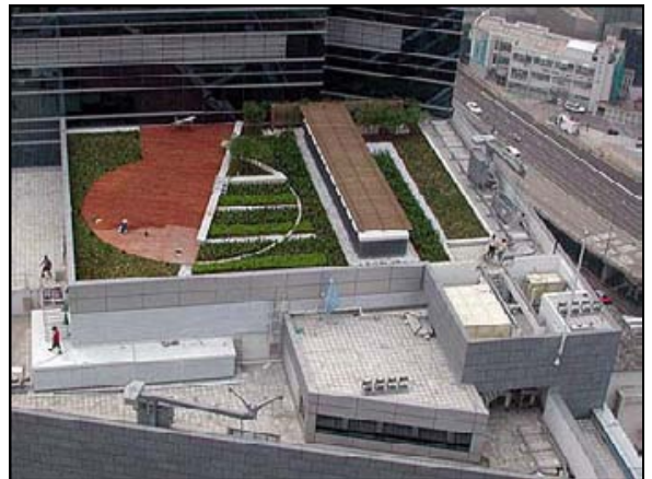
2.2 – New Police Headquarters (Wan Chai District) (Source and copyright © by ArchSD)
