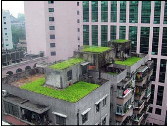
Figure 3.12 Site B – Guang Wei Lu Residential Buildings
