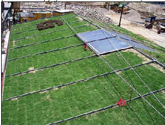
Recent photos showing one side covered in lawn and the other left to its own resources. (Source and copyright © Gammon-Skanska, 2006)
