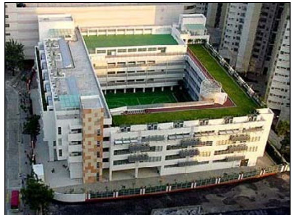
7.2 – Primary School at Sze Mei St. San Po Kong (Wong Tai Sin District) (Source and copyright © by ArchSD)
