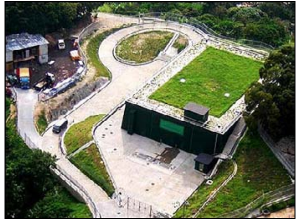
4.3 – Wah Fu Fresh Water Service Reservoir (Southern District) (Source and copyright © by ETWB)
