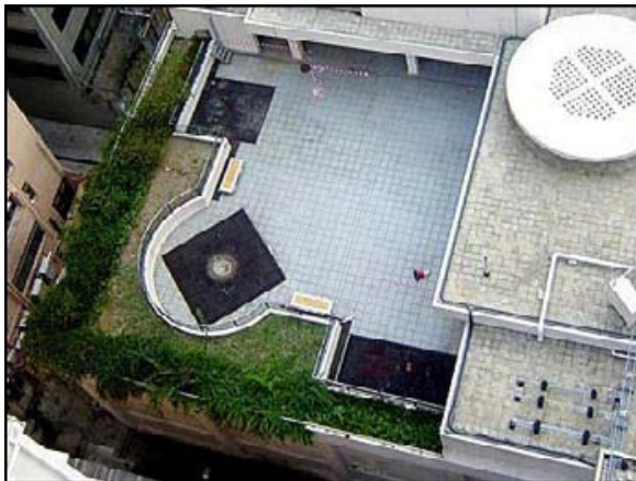
2.1- Bowrington Road Market Roof-top (Wan Chai District) (Source and copyright © by Urbis 2006)
