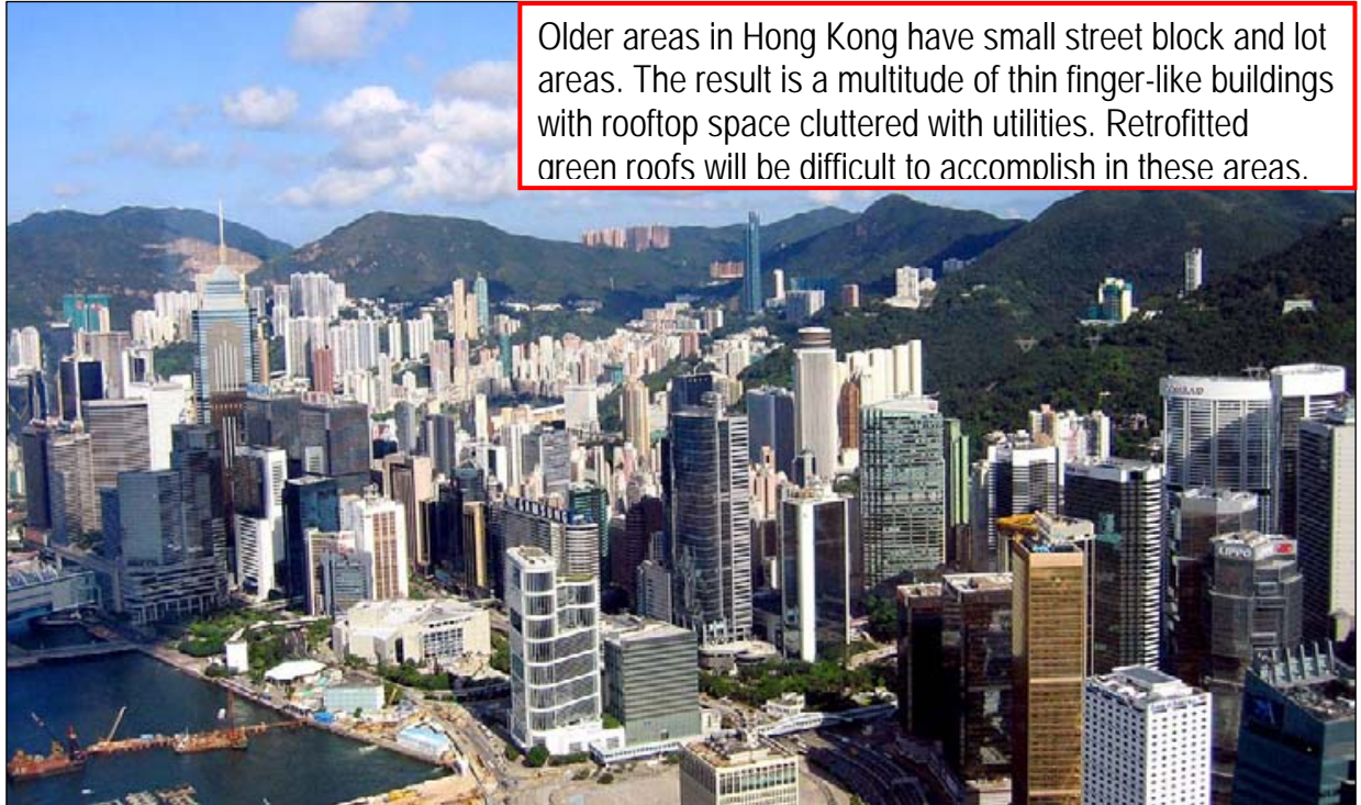
Views from IFC, Central, looking East Towards Wanchai, Hong Kong Island (Source and copyright © 2006 Urbis Ltd.)
