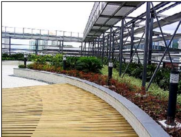
6.9 – Education Resource Centre cum Transport Interchange (Kowloon City District) (Source and copyright © by ArchSD)
