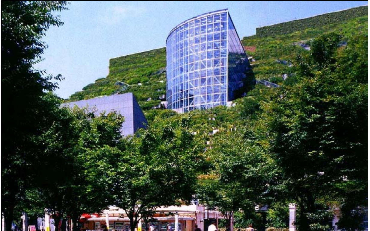
Figure 3.4 Intensive Green Roofs on the ACROS Office Block Building, Fukuoko, Japan
