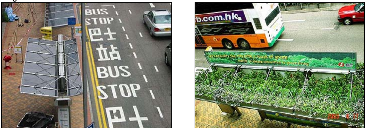
Before and After (June 2003) photos of bus shelter green roofs experiment in Causeway bay. (Source and copyright © John YAU (Chun Wang), 2003)
