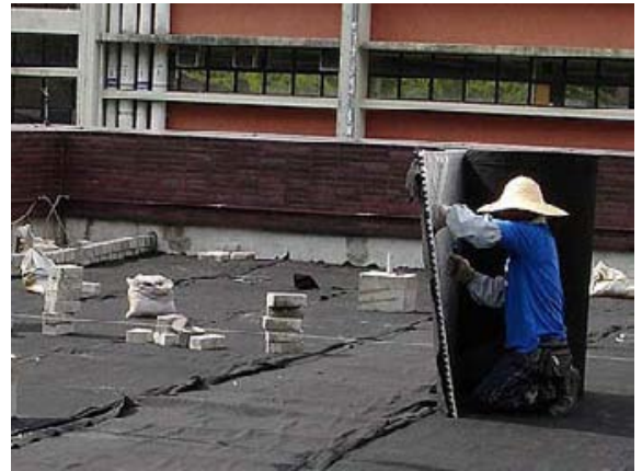
Drainage layers being installed at HKU (Source and copyright © Cheung Shing Yuk Tong Co. Ltd., 2006)
