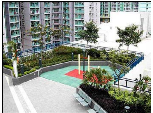
18.4 – Tseung Kwan O Area 73A, Phase 1 (Sai Kung District) (Source and copyright © by Housing Dept.)
