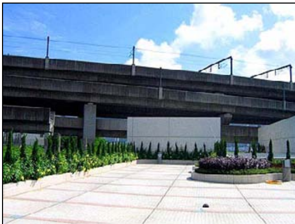
10.11 – Public Mortuary at Area 26E (Kwai Tsing District) (Source and copyright © by ArchSD)
