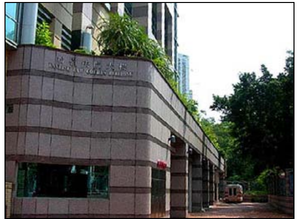
16.3 – Fanling Magistracy Building (North District) (Source and copyright © by ArchSD)
