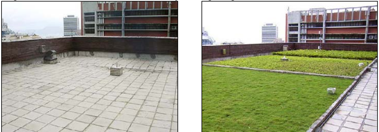
Before (June 2006) & After (August 2006) photos of experimental green roof at University of Hong Kong. (Source and copyright © Cheung Shing Yuk Tong Co., Ltd., 2006)
