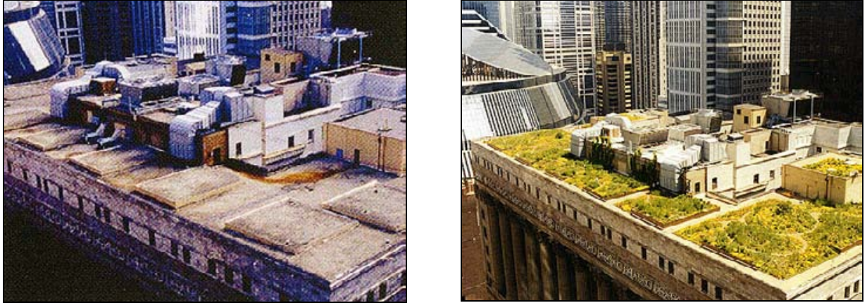
Views showing the City Hall building before and after the addition of extensive rooftop gardens. (Source and copyright © Earth Pledge, 2005)
