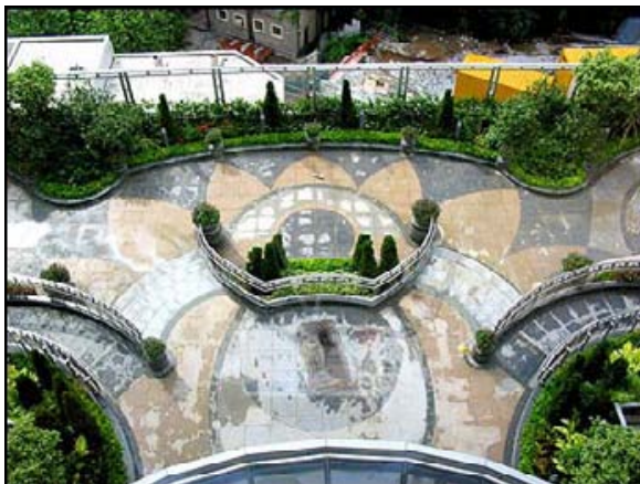
6.1 – Kowloon Hospital (Kowloon City District) (Source and copyright © by ArchSD)
