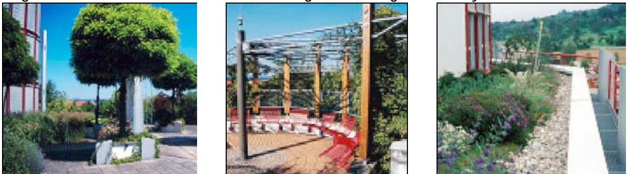
Figure 3.2 Intensive Green Roof, Lauer Building, Unterensingen, Germany
