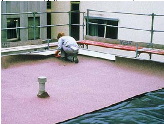
Protection layer/moisture retention mat being installed above the waterproofing/root barrier in Europe. (Source and copyright © Greenlink Küsters Ltd.)
