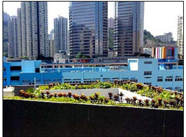
10.10 – Kwai Chung Ambulance Depot (Kwai Tsing District) (Source and copyright © by ArchSD)
