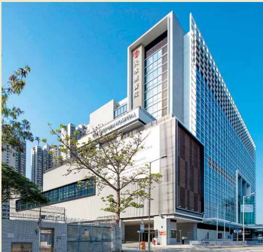
Design-and-Build Project – Tin Shui Wai Hospital
