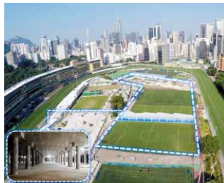
Happy Valley Underground Stormwater Storage Scheme
