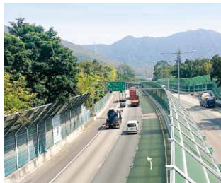
Retrofitting of Noise Barriers on Fanling Highway
